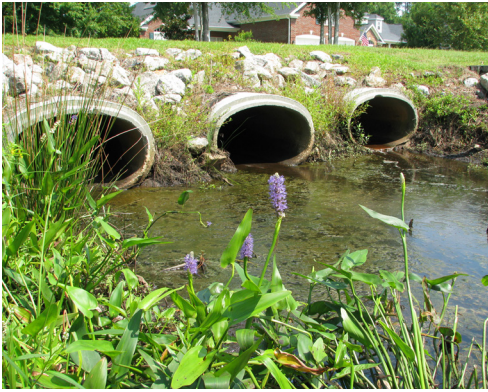
Inlet pipes convey stormwater from paved surfaces to the pond.
